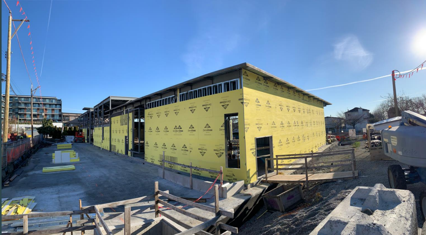
Structural steel studs & sheathing
