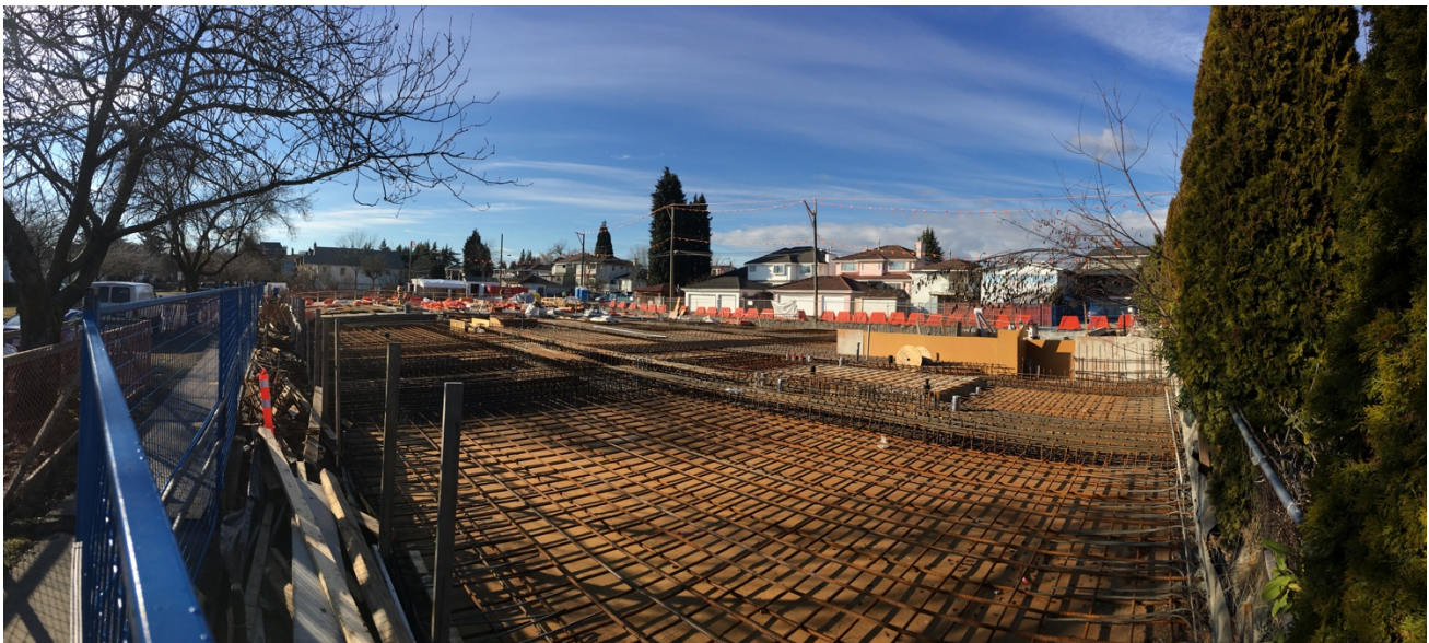
Picture 8: View from the south-east corner of the property (March 08 2019)
