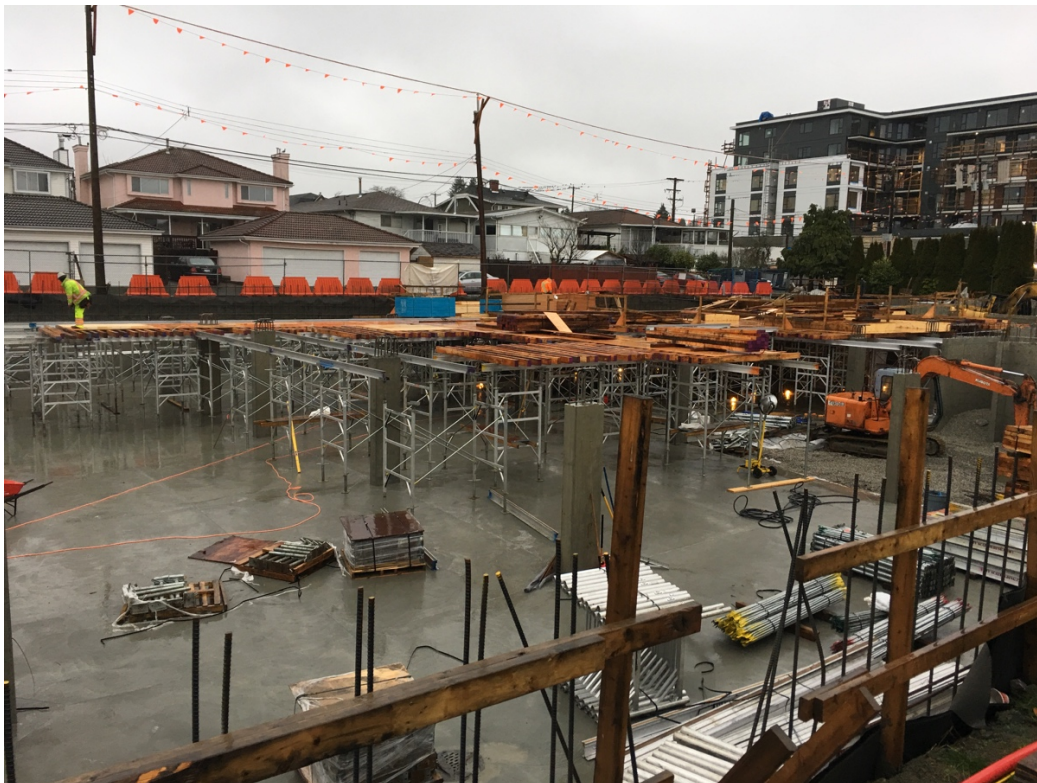
Picture 2: The underground parking (January 03 2019)
