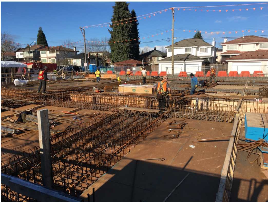
Picture 4: Rebar work (February 02 2019)
