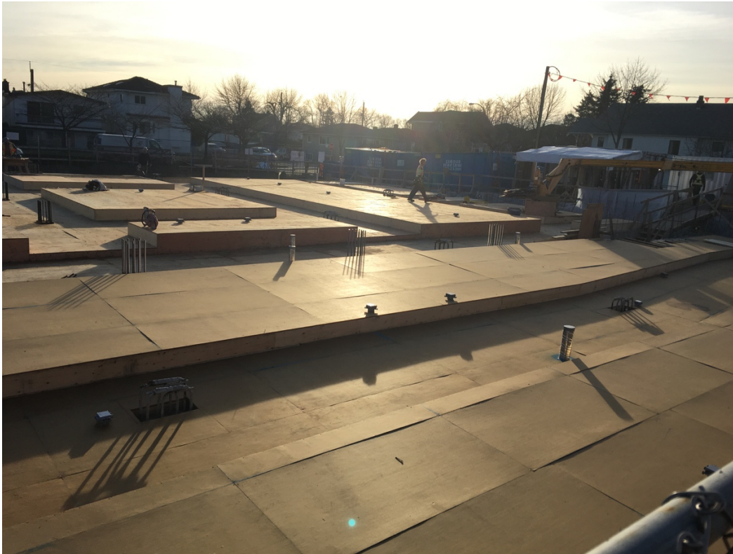
Picture 3: Formwork (January 21 2019)
